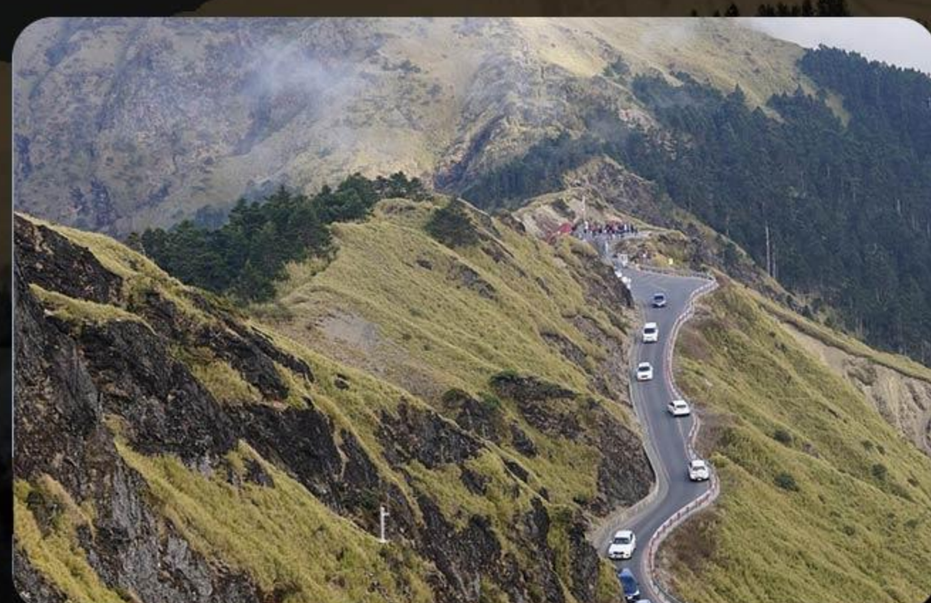
Safety Monitoring of Slopes Along Highways
