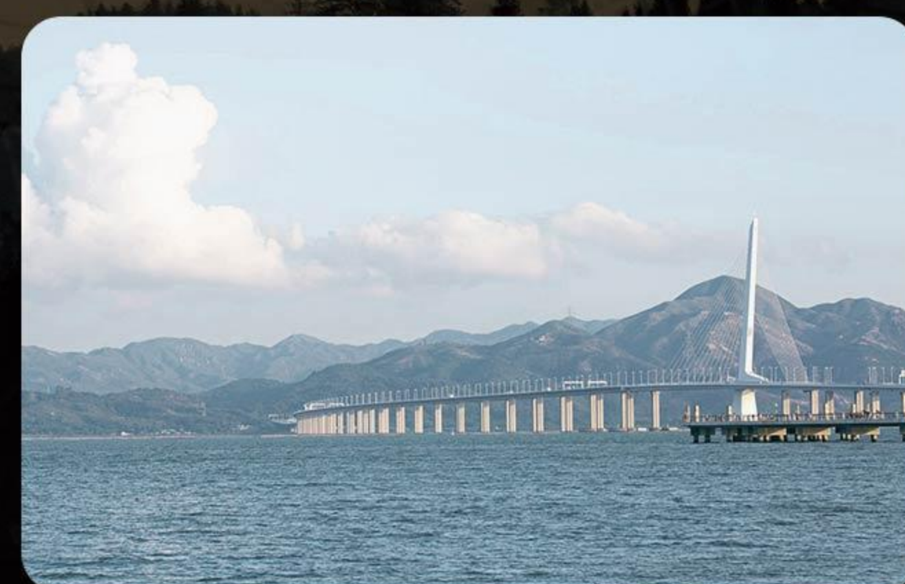
Bridge Structure Monitoring
