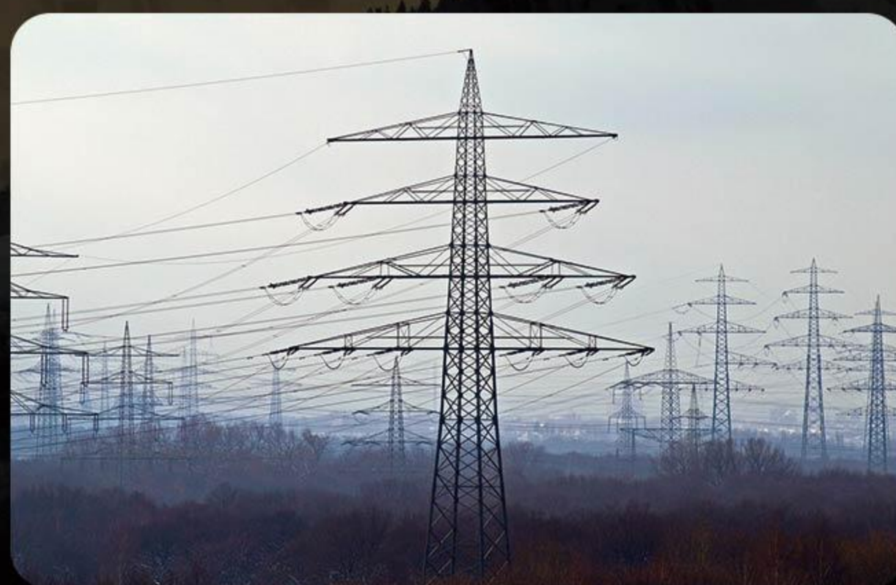
Power line surveying
